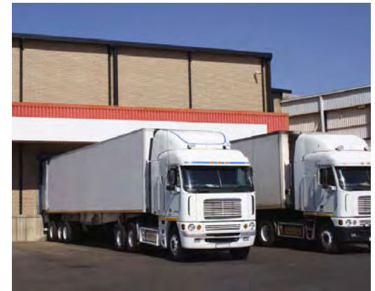
Loading bay of large cold store
